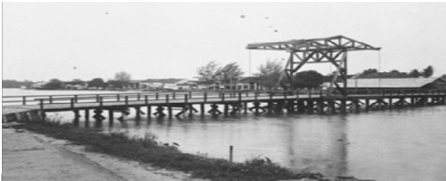
The photograph shows a lift bridge over the Silau River in Tanjung Balai The photograph was taken between 1900 and 1916 (A collection of Tropen Museum by a photographer named C.J. Kleingrothe).
