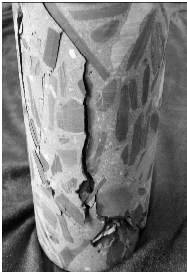
Figure 3: Failure Mode of Ordinary Concrete in Compression
