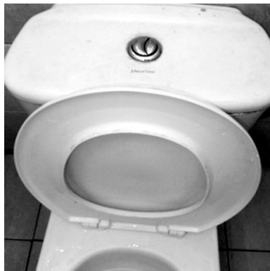
Figure 3: The use of water cistern with dual flushing system for toilet in WAKAF TEMBESU MOSQUE, TERENGGANU Source: Field work March 2015
