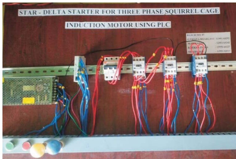
Figure 2: Hardware Setup with PLC
