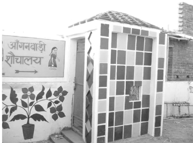
Toilet in Anganwadi
