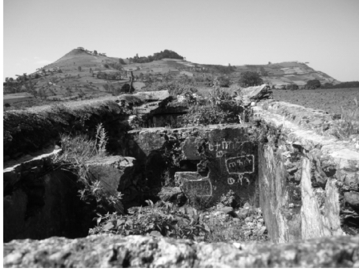
Figure 14: Part of the ruins of Emperor Suseneyos's palace at Aringo Abo
