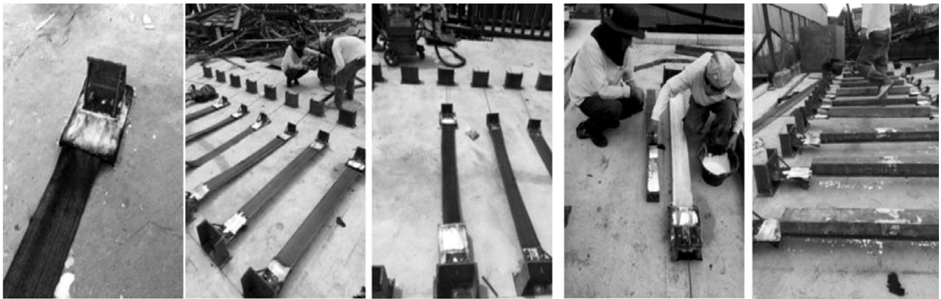
Figure 2: Process of timber beam strengthened by prestressing CFRP sheets
