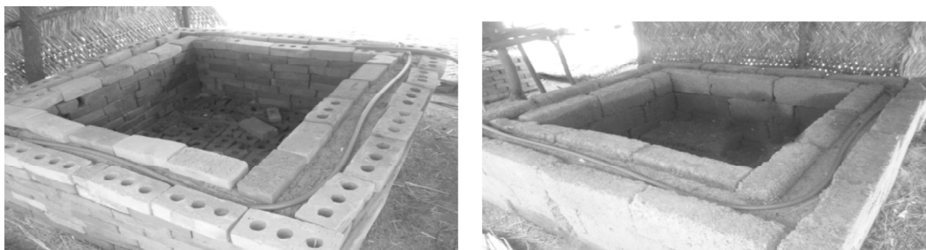
Figure 1: Fired brick (left) and Mud block (right) Zero Energy Cool chambers
