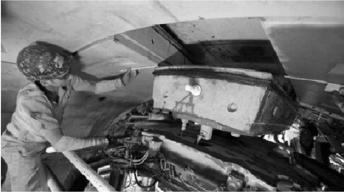
Figure 2: Application of pre-cast segments
