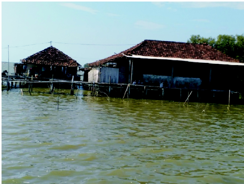
Figure 4: House Stage: increasing elevation of the floor in the village Bedono
