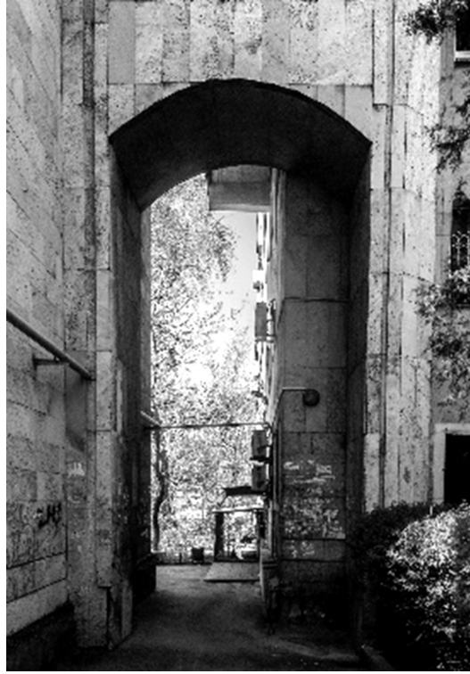
Figure 8: The arch separating the internal space from the external space
