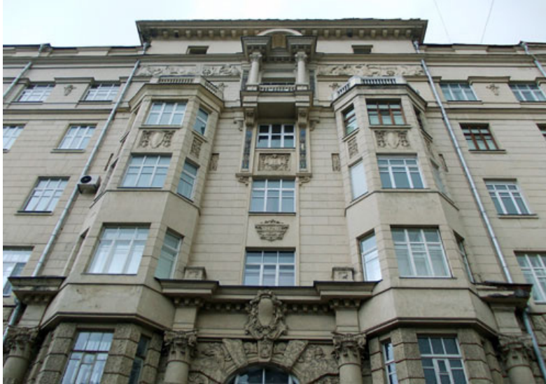
Figure 1: 20 Povarskaya Str., Moscow– a monument of architecture of the XXth century, included into the UNESCO catalogue
