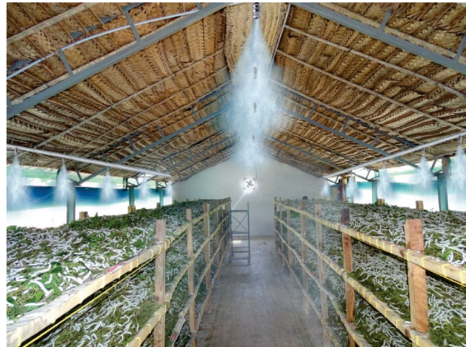
Design of fogging system in silkworm rearing house
